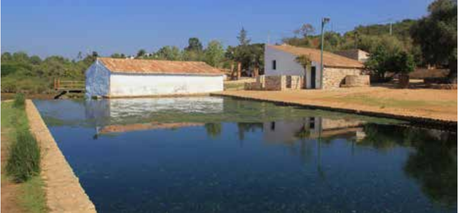
Dam, tide mill and the old miller's house
